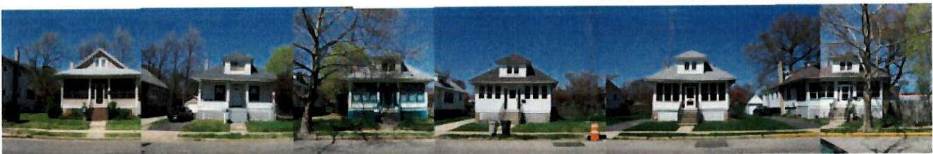
Figure 2.16: North side of Progress Avenue - Tatum to North Broad Streets
