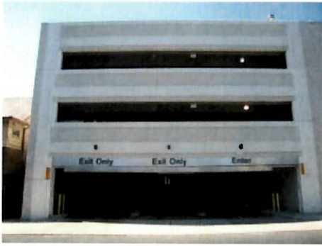
Figure 3.2: Entrance to the County parking garage on Cooper Street
